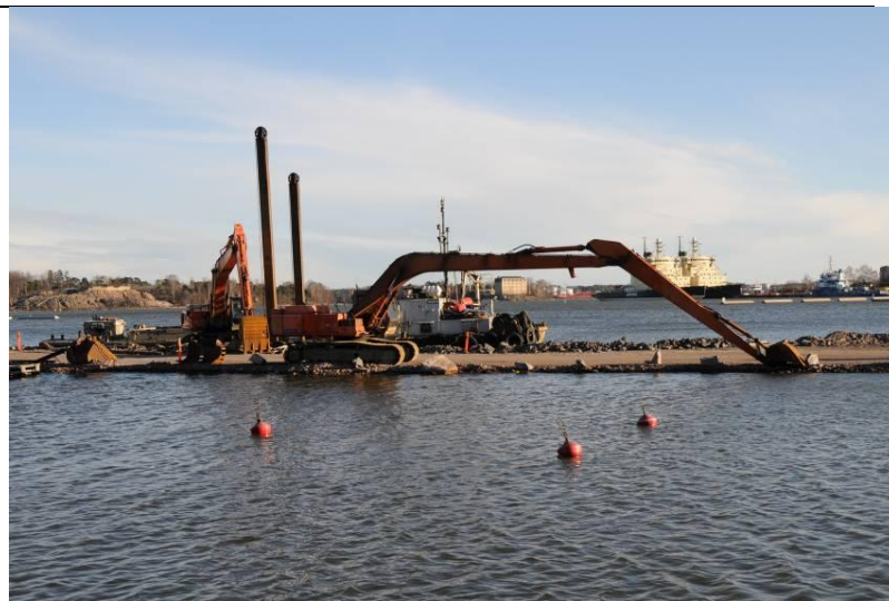
Figure 95 A dredger at work in near Helsinki, Finland. (Photo: Metsähallitus)
